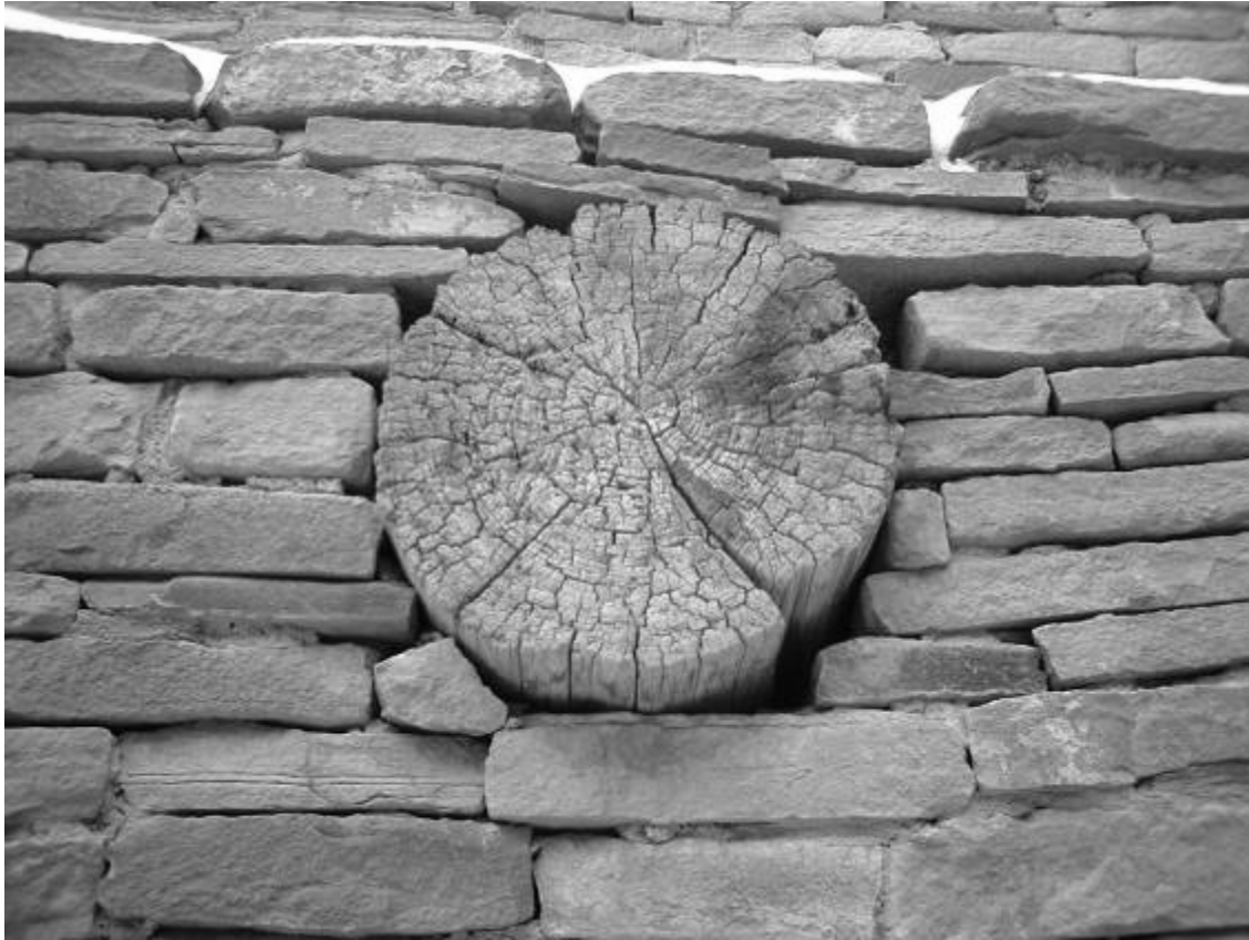
Figure 7. 11 Cross section of a primary beam. Crosssections from the main support beams can be sampled to collect a complete series of years. Cutting dates can be obtained by cross dating the ring series of these dead trees against a master chronology of the area to assign exact felling dates, demonstrating when the trees were cut for incorporation into the architecture (photo by Jim Speer).
